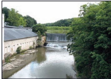
The project provides the public with scenic views of the Chagrin River from Cleveland and Main streets and complements redevelopment plans for a closed paper mill.
